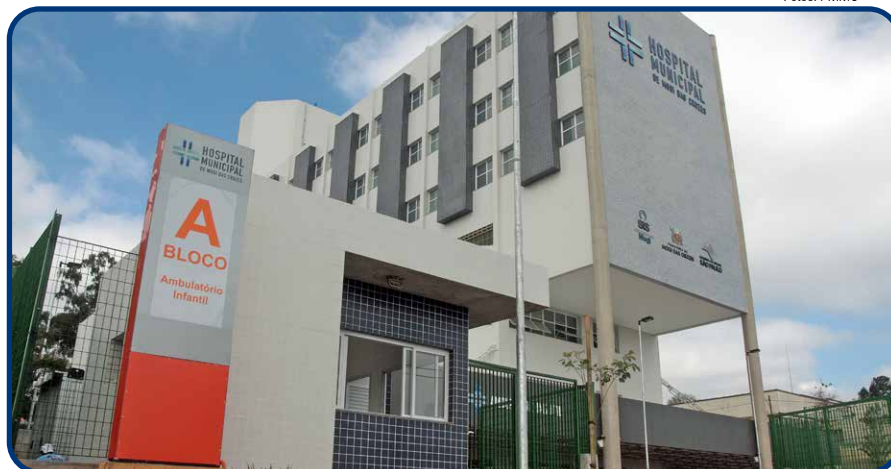
Fachada do Hospital Municipal de Mogi das Cruzes
