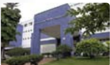
Hospital Municipal de Osasco
