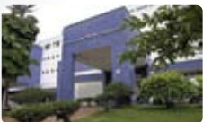
Hospital Municipal de Osasco
