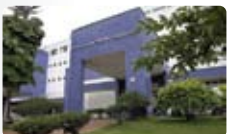
Hospital Municipal de Osasco
